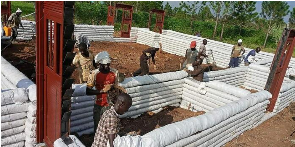
Figure 1: Builders constructing a house in Kenya using earth-bags (Austin, 2023)
